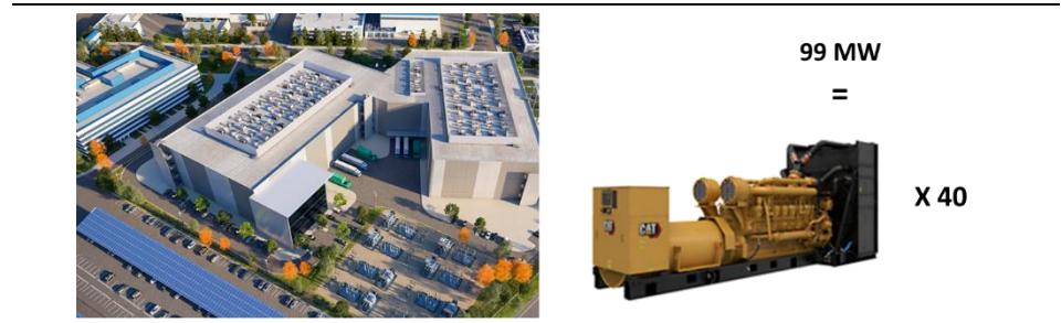
Fig. 161: Edgecore Internet’s data centre with 99 MW diesel backup
